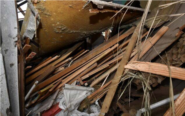
The flags were found in the collapsed storeroom at Kibbutz Be'eri, southern Israel, on December 6, 2023. (Sarit Uziely)
